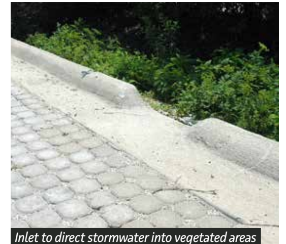
Vegetated landscape islands in parking lots provide infiltration areas for rainwater
